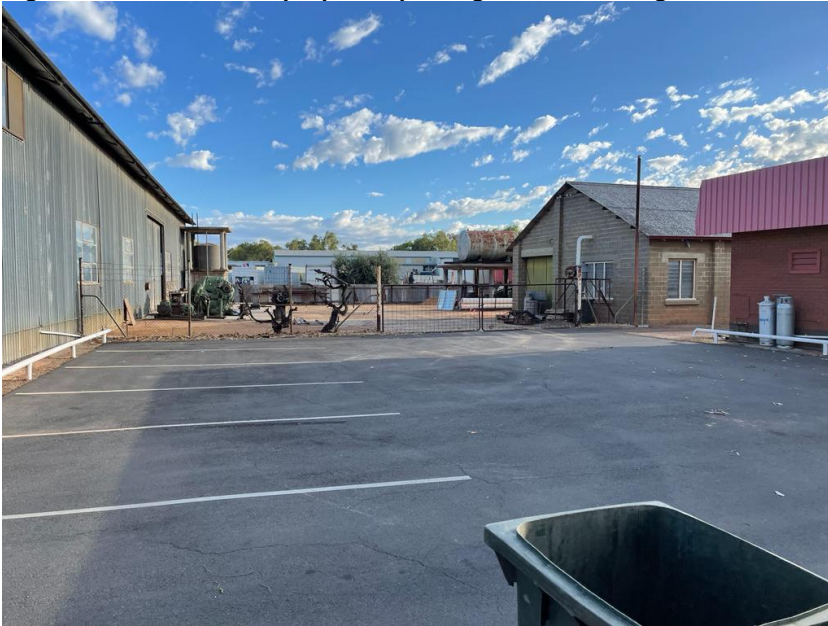
Figure 3 – View towards proposed parking area, screening to be installed along fence and gate
