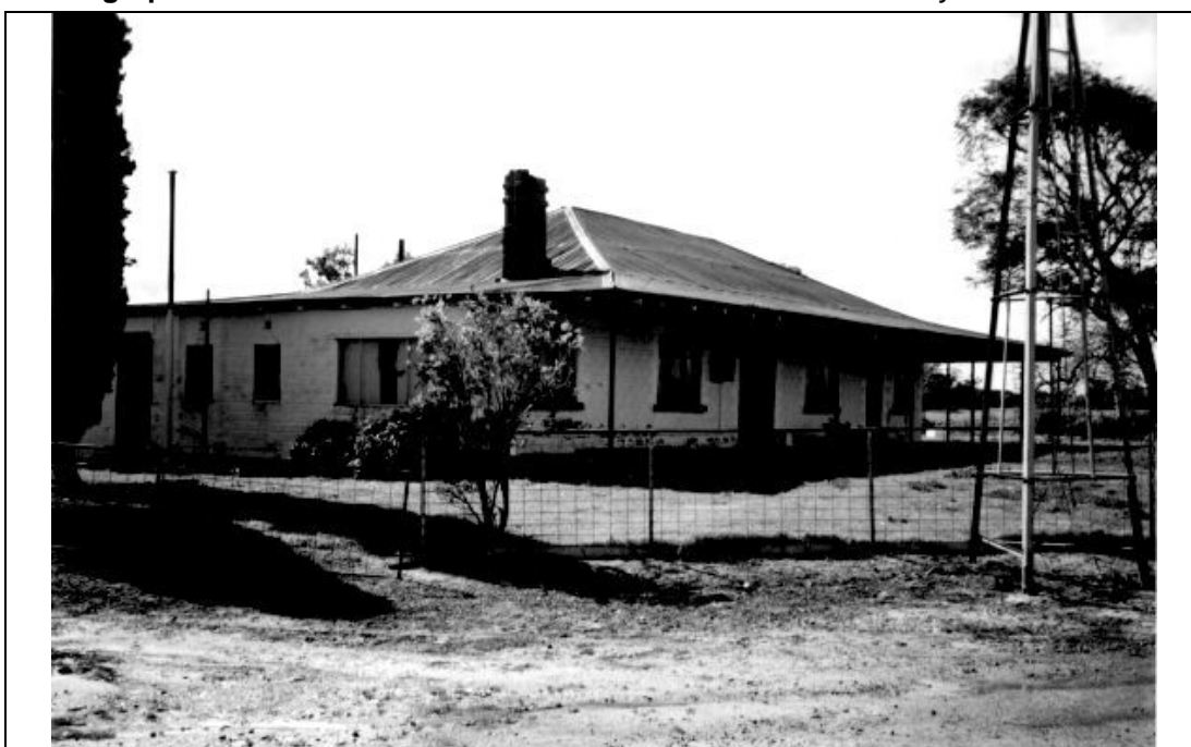
South west facade, Shady Grove Homestead
