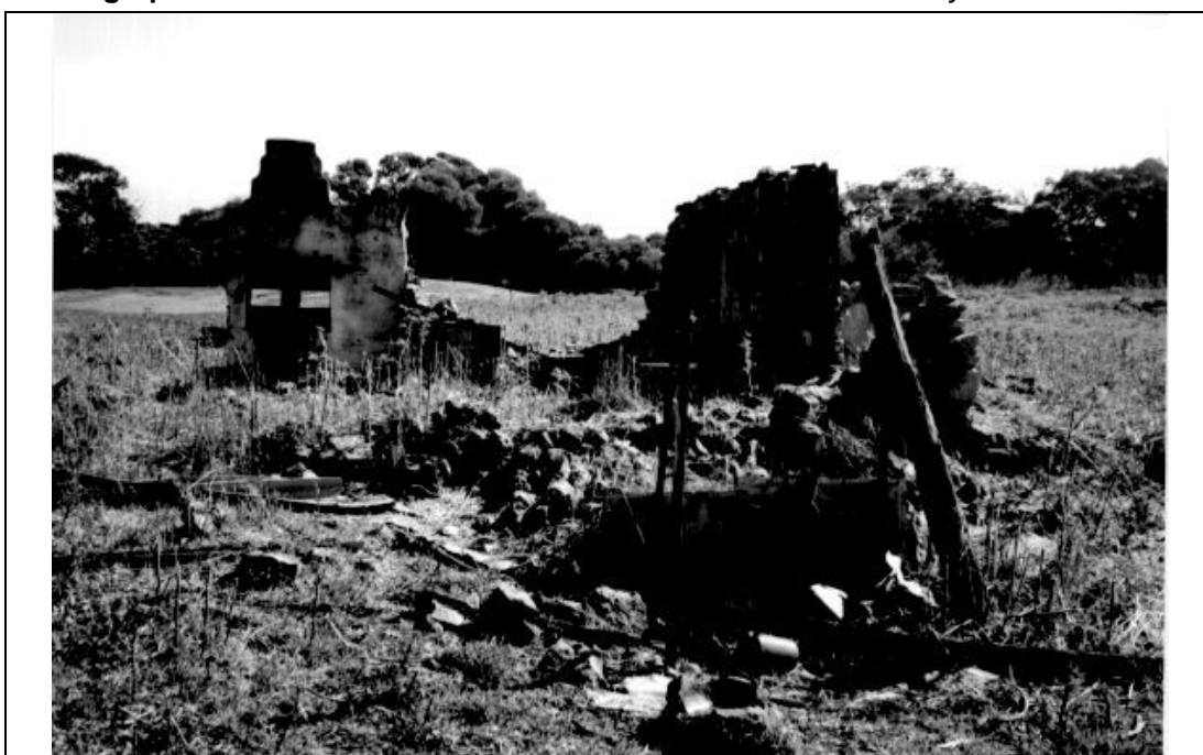
View of ruin looking north
