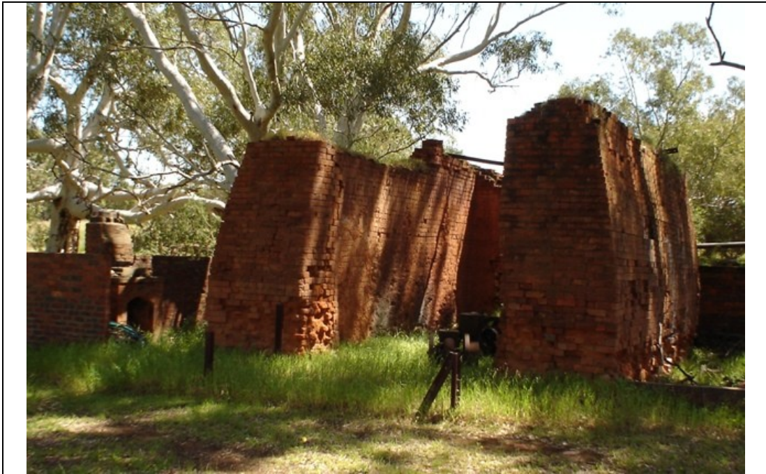
Kiln, looking north
