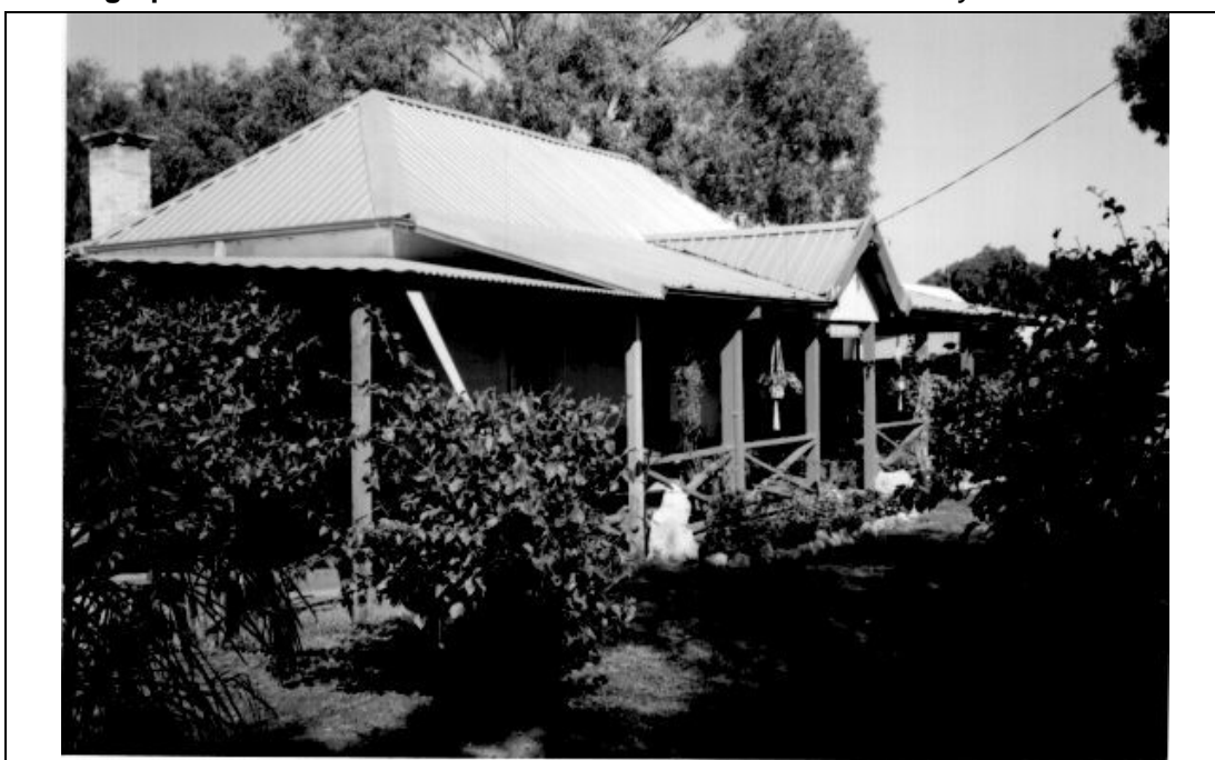
Peppercorn Cottage, north facade
