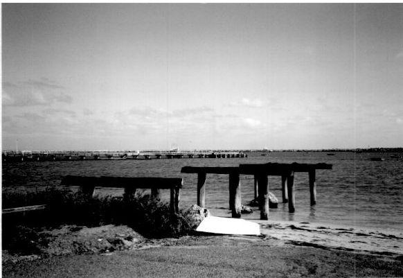
Remains of jetty, looking south east.
