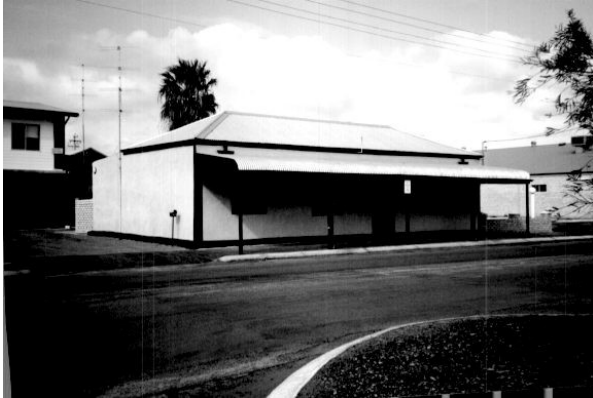
Front façade facing Pt. Leander Drive
