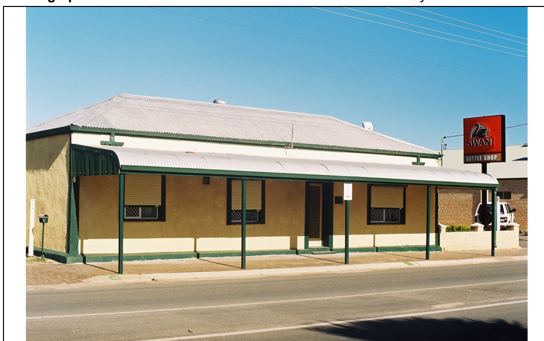
Front façade facing Pt. Leander Drive
