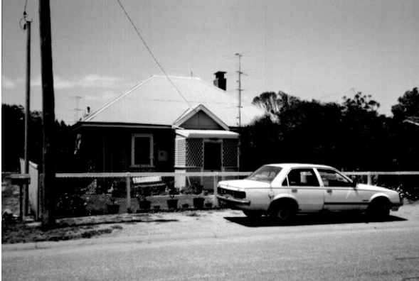
West (front) side of house from Hepburn Street
