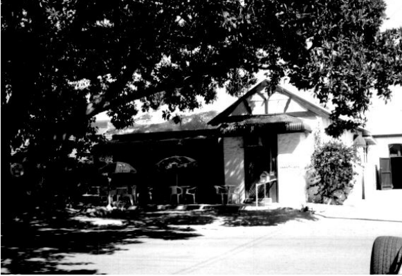
Front (North) aspect from Moreton Terrace
