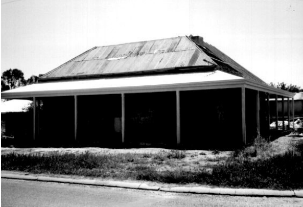
Southeast aspect during reconstruction
