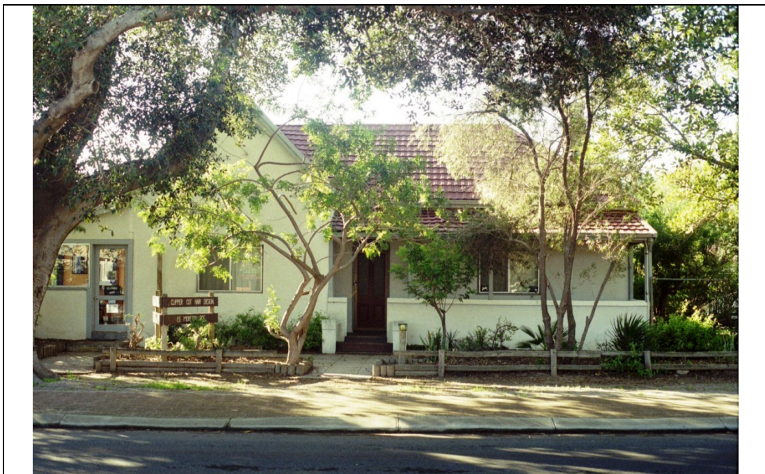
Front facade from Moreton Terrace
