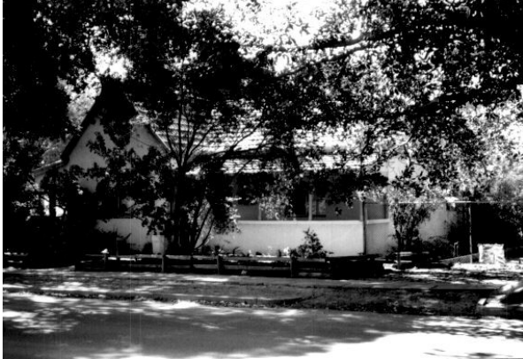
Front façade from Moreton Terrace
