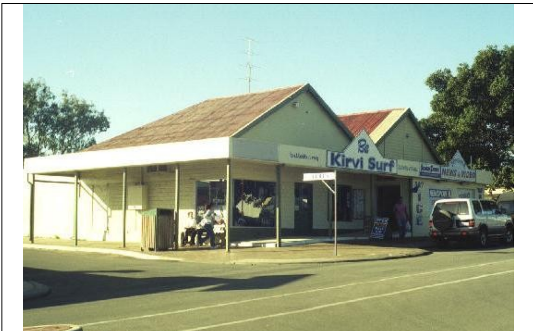
View of the south west façade.
