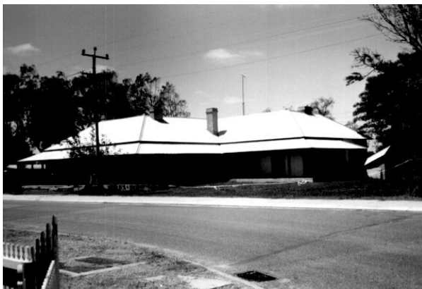
View from Hunts Road looking south-east
