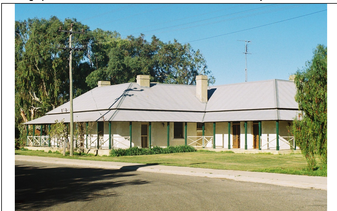
View from Hunts Road looking south-east
