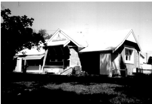
Library, former Post Office, east elevation
