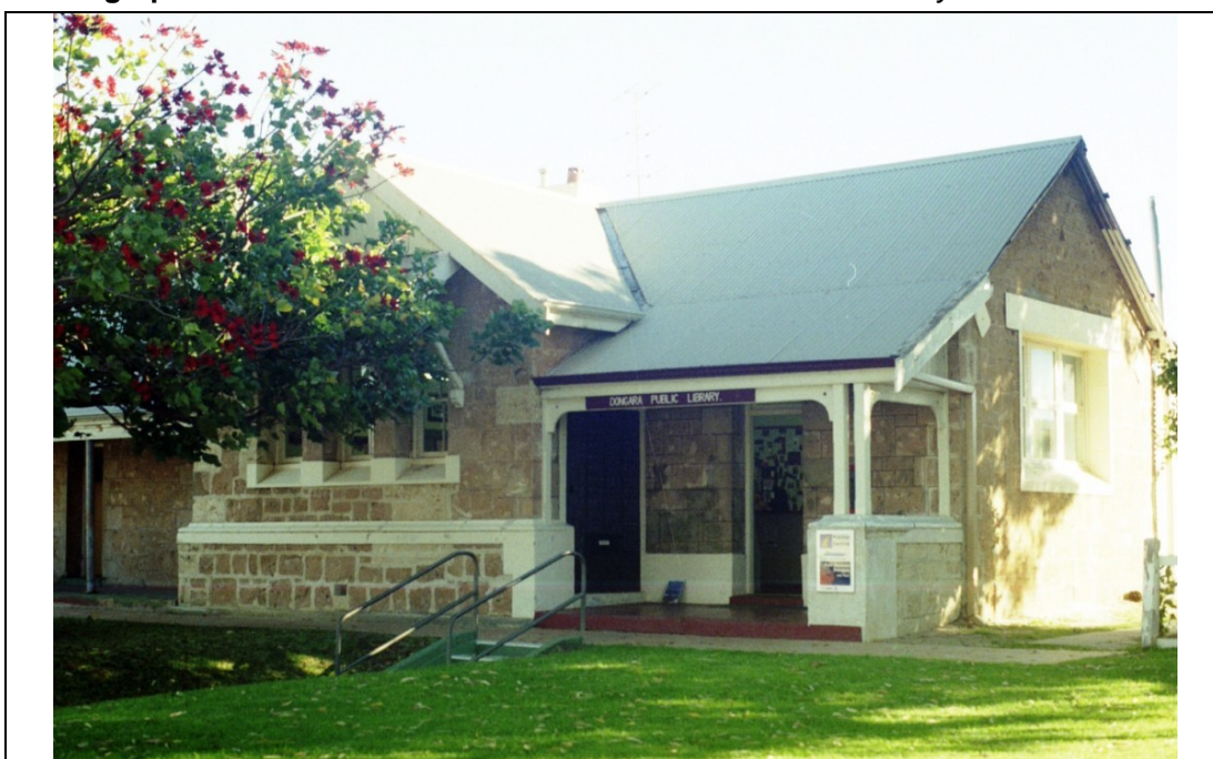
Library, former Post Office, east elevation
