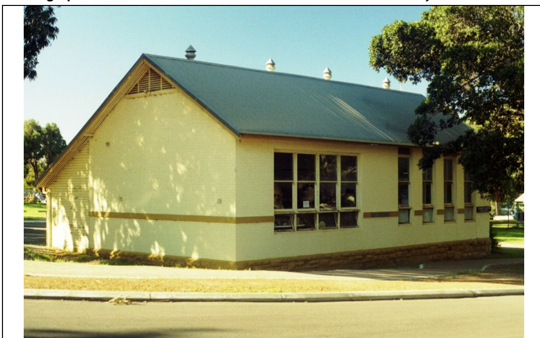
Dongara Second School, south and west facades
