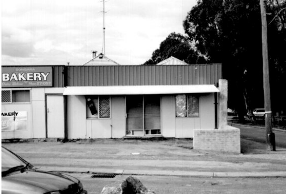
West facade viewed from Waldeck Street
