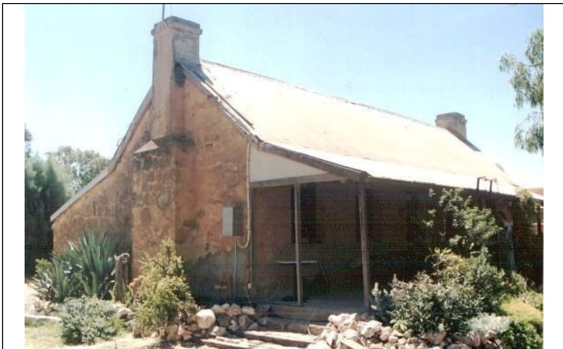
Former Catholic Presbytery, south and east elevations
