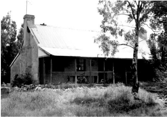
Former Catholic Presbytery, south and east elevations.
