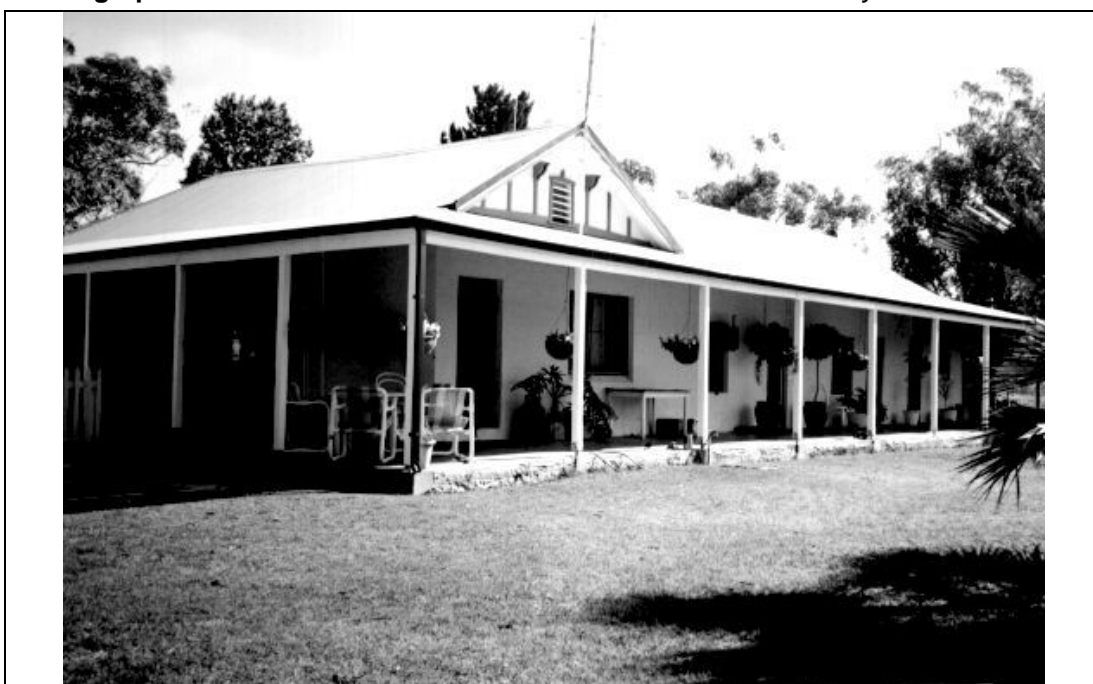
View of the east facade.
