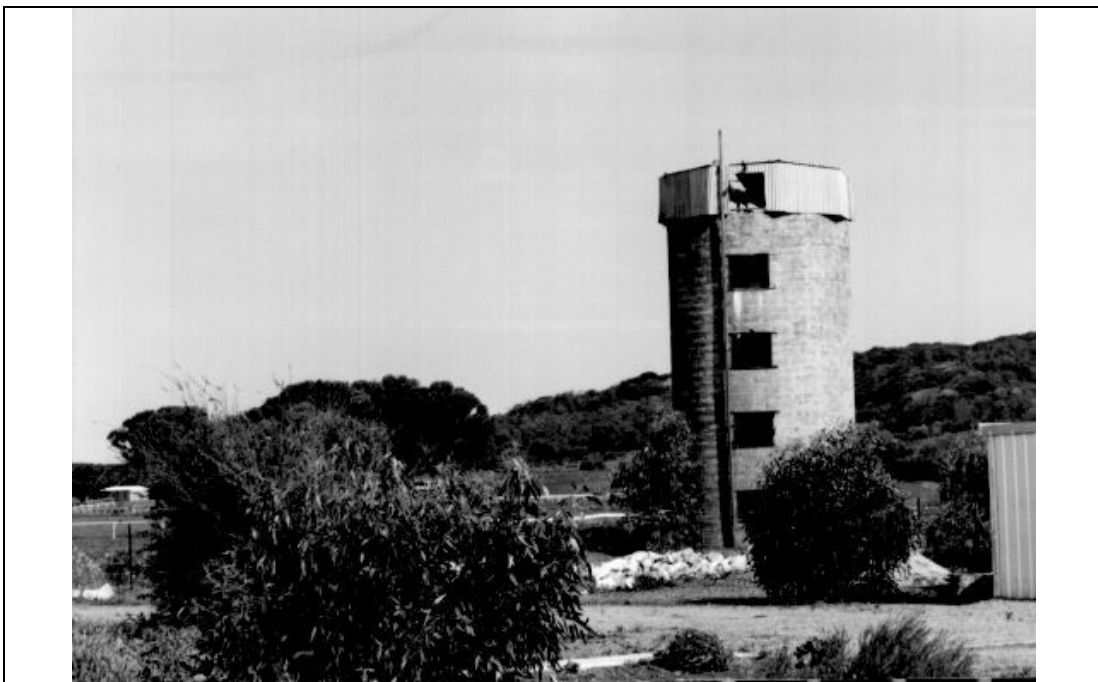
Silo, east elevation
