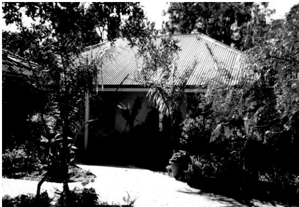
Bonniefield, west façade
