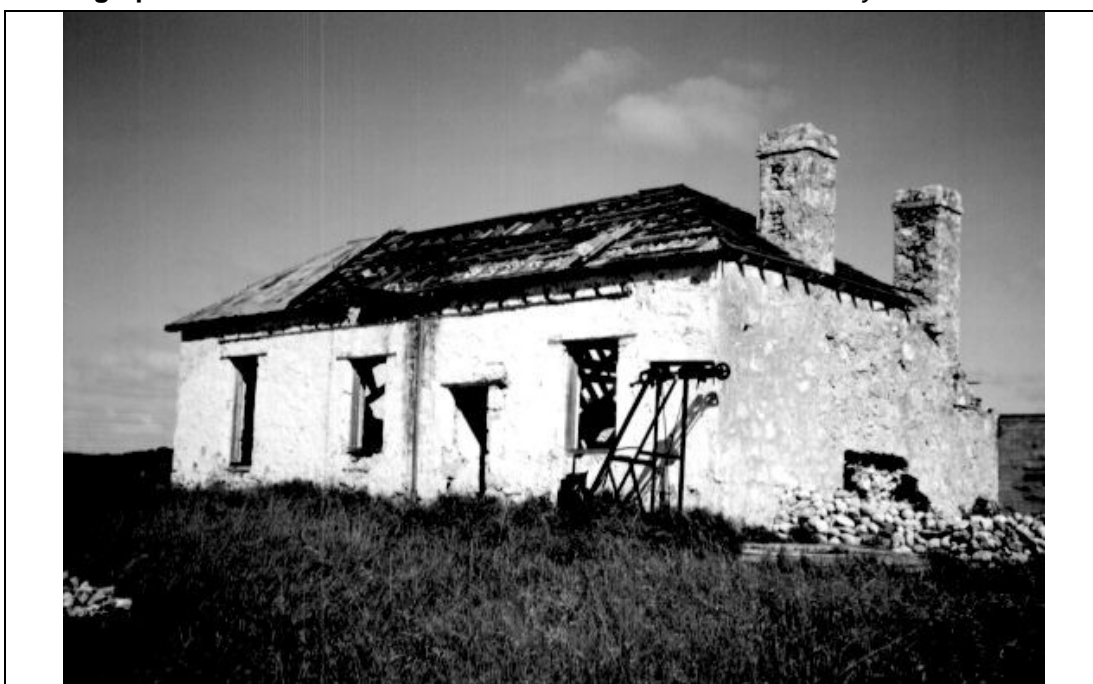
Nhargo Farmhouse, east elevation.
